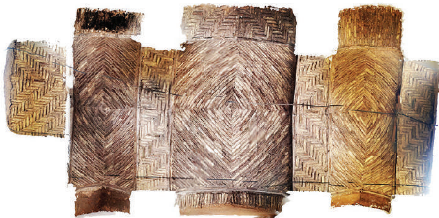
Orthoimage of the Brickwork of the Vaults and Domes Seen from Below
